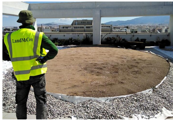
Roof garden construction at National Bank of Greece, Moschato
